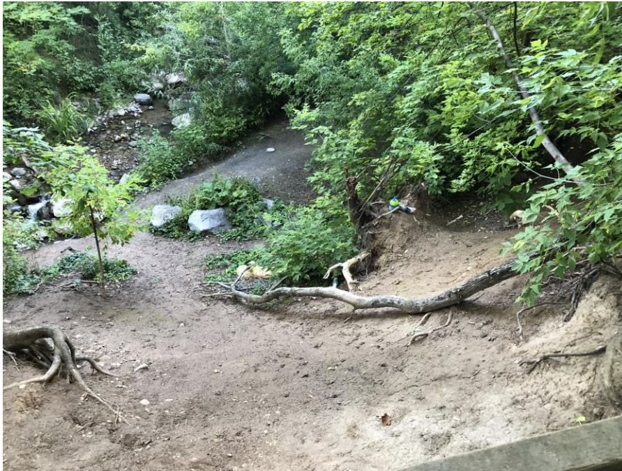
Photo #11 – Erosion that has occurred from sprinklers and runoff from neighboring properties
