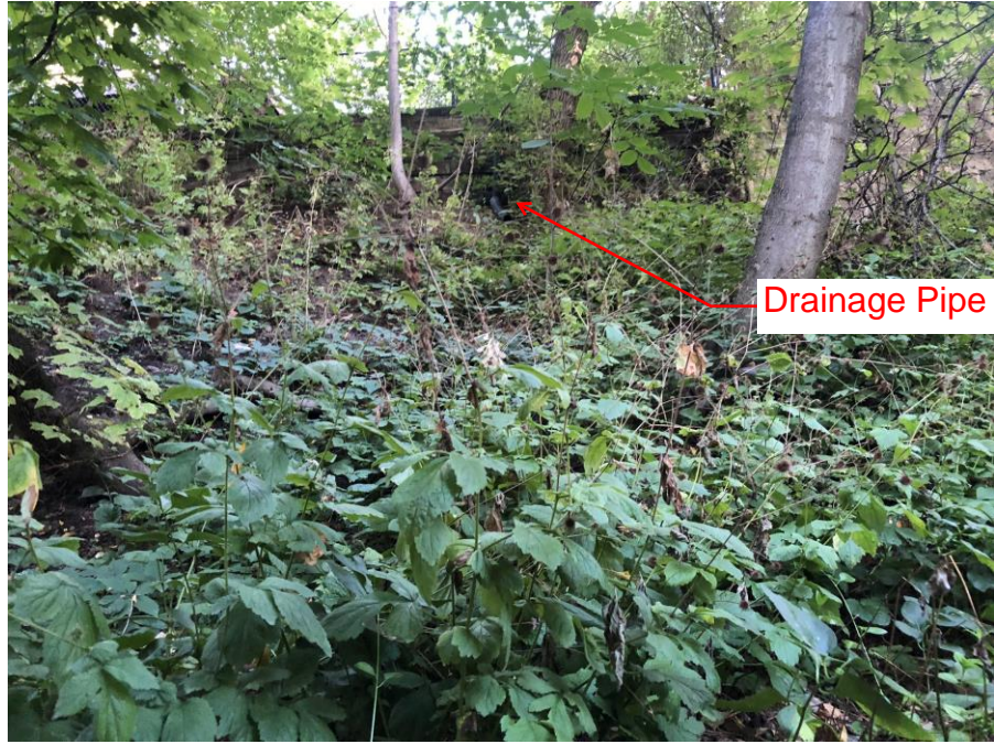
Photo #5 – Image of drainage pipe from neighboring property owners
