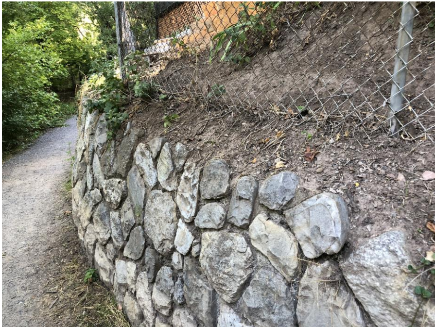
Photo #14 – additional soil has been added above the wall and should be removed
