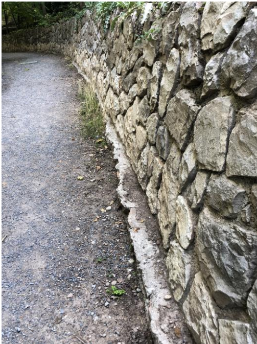
Photo #6 – Image of drainage pipe from neighboring property owners, example of adjacent structures encroaching on the existing rock walls, and example of toe of retaining wall being undermined.
